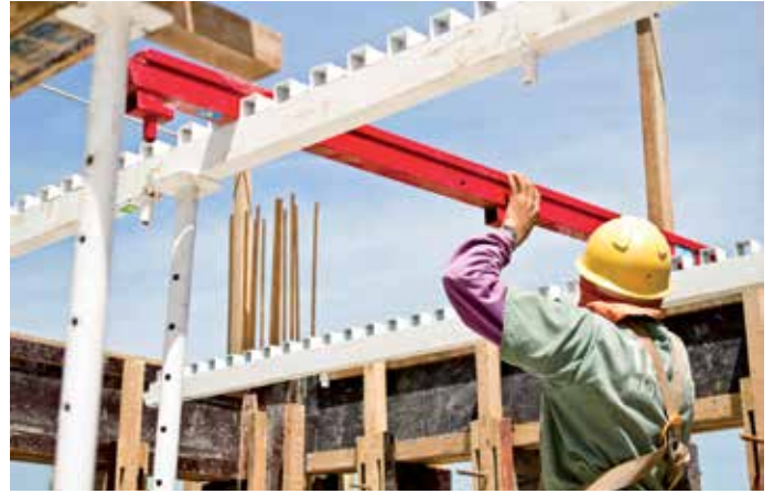
The system consists of two basic elements: Multiple notch stringer and Joist.
