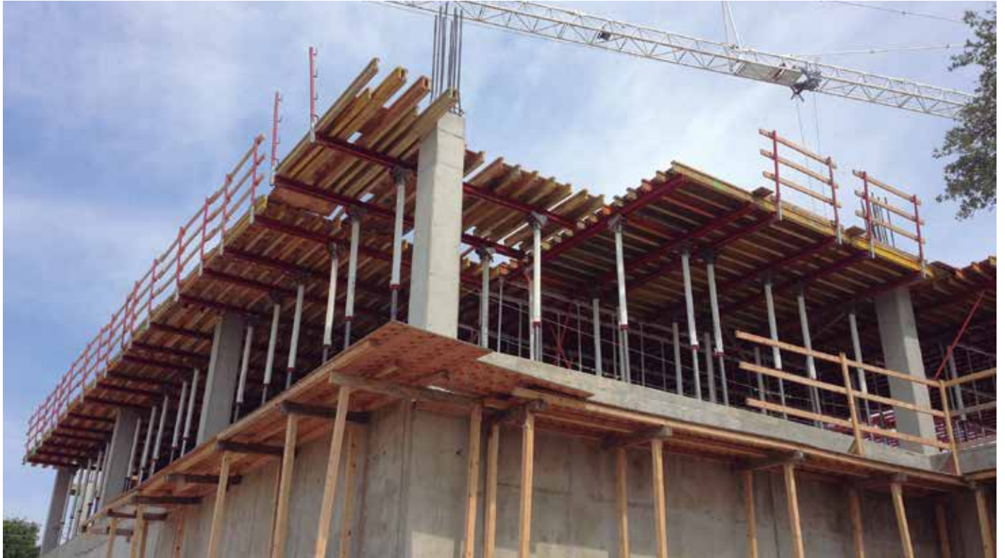
Rollingwood office building, United States
