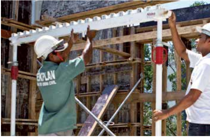
The metal joist is the element that is used most frequently, therefore it is lightweight and resistant.
