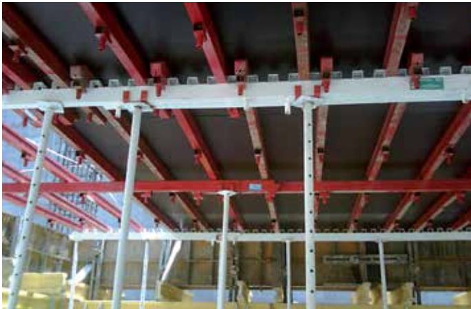
The system's structural elements, the stringer and the Joists can be overlapped in both directions or butted instead (built-in secure connection).
